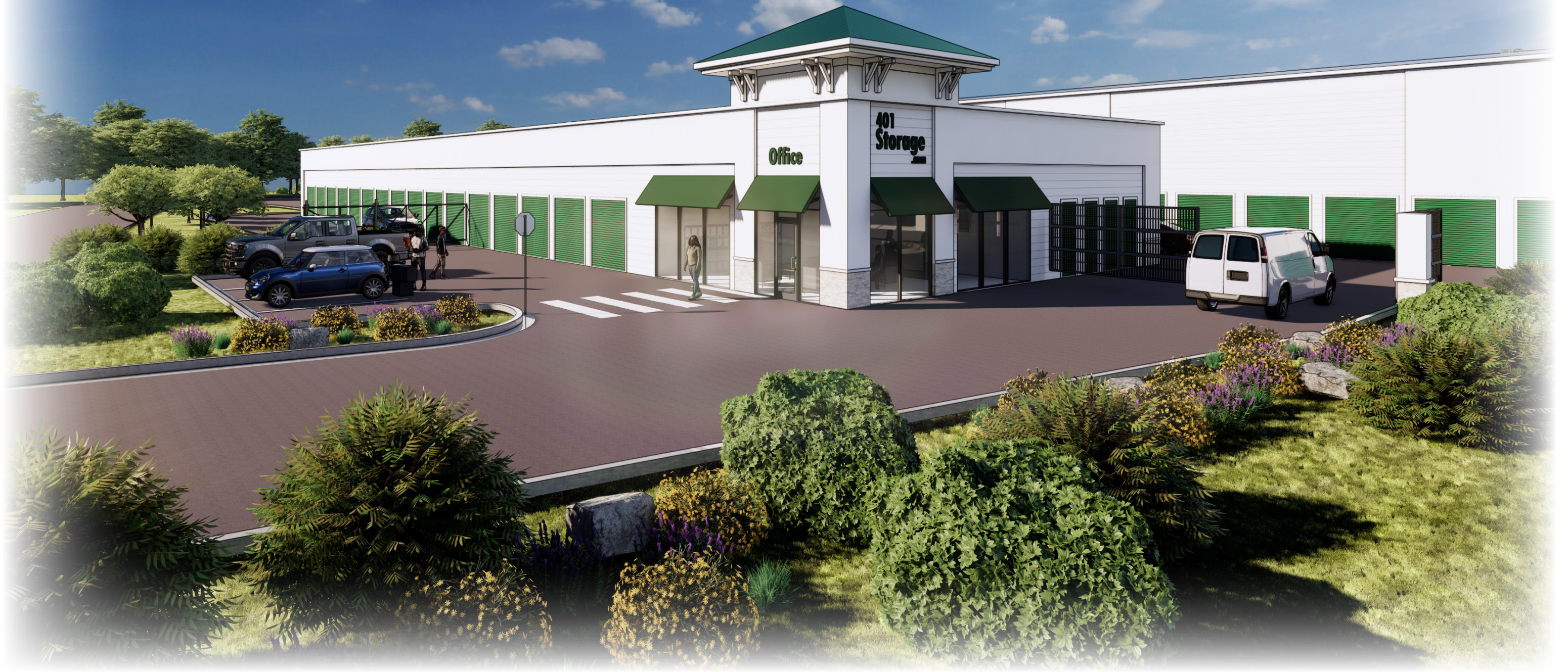
BUILDING A- OFFICE VIEW
